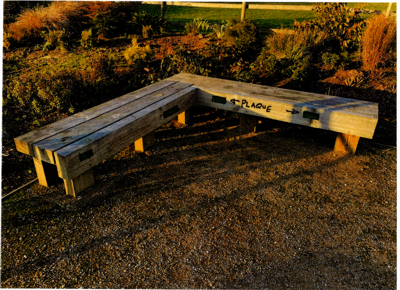
Typical example of a bench constructed from railway sleepers
